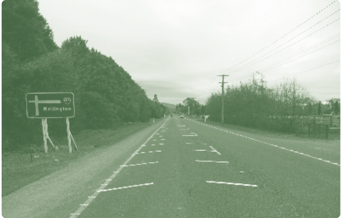
The field trial site on State Highway 57
