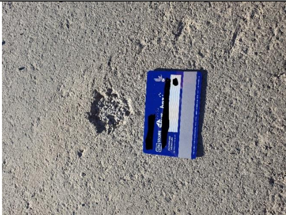
Small 'pop-outs' showing the solid layer below.
