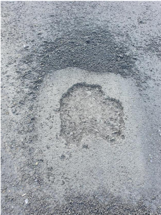
Small 'pop-outs' showing the solid layer below.
