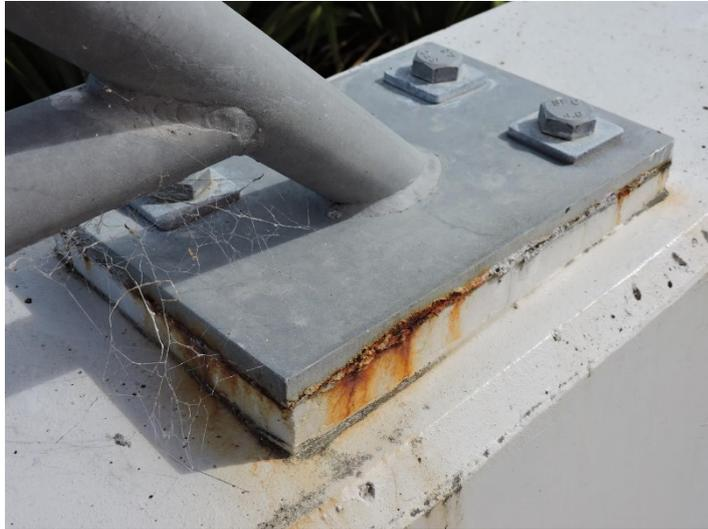
**Figure 10.8:** Example of the condition of the underside of the baseplate
