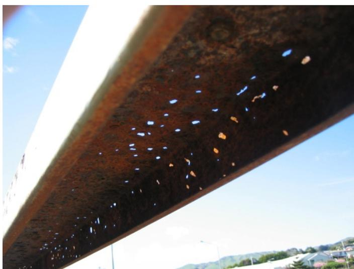
**Figure 10.6:** Unpainted galvanized base plate of handrail on coastal bridge
