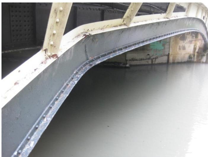
**Figure 6.4:** Example of damaged coatings - Auckland Harbour Bridge
