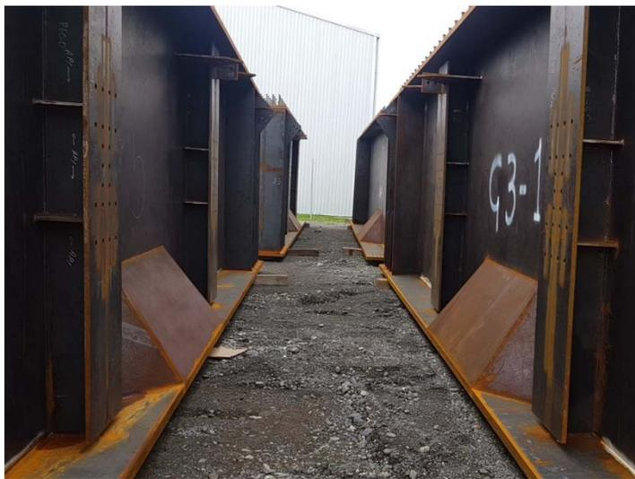
**Figure 5.3:** Example of flared stiffener on bridge girder to discourage climbing
