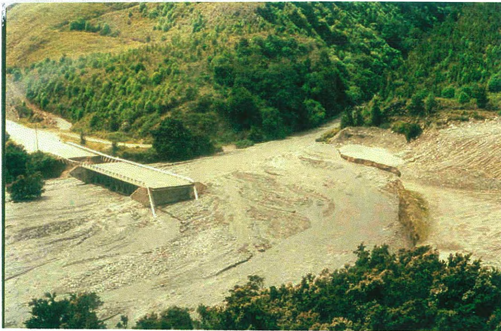
Figure B6. Sediment build-up filling the channel to the base of the bridge superstructure; flow is to the left (from Melville & Coleman 2000).
