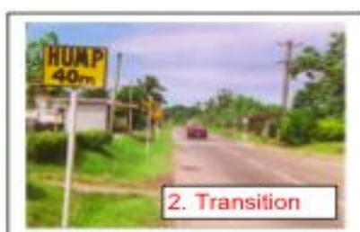
The carriageway width is reduced from 7.3 m to 6.5 m. Shoulder width increases from 1.5 m to 1.9 m. Signing is normally placed before the physical restriction and rumble strips can also be added.
