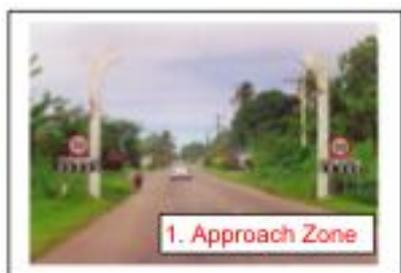
Drivers are made aware that speeds must be reduced from 100 km/h to 50 km/h. This is done by adding a gateway and a road marked bar pattern (17 bars) can also be added in front of the gateway.
