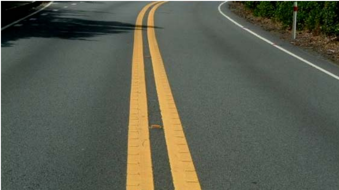
Figure 3.2 ATP Double yellow centreline on two lane road with ribs on outer edge only. Edgelines are non ATP.
