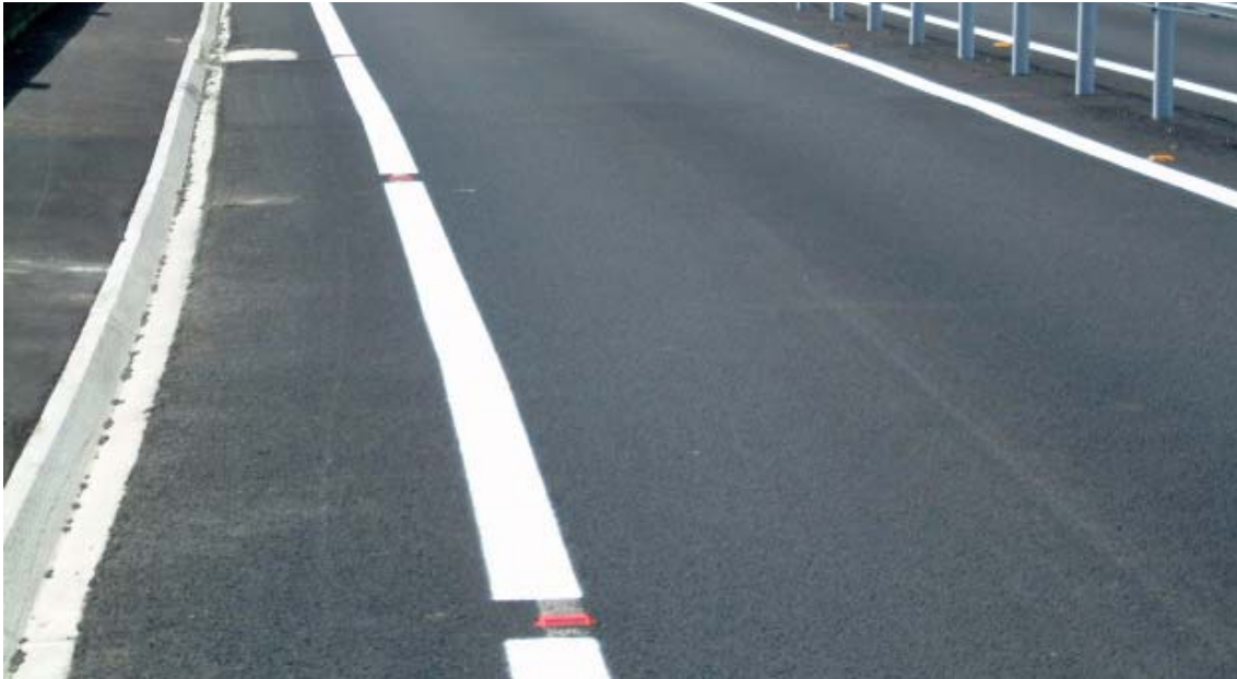
Figure 4.2 A situation where ATP edge-lines could be considered in association with a safety barrier
