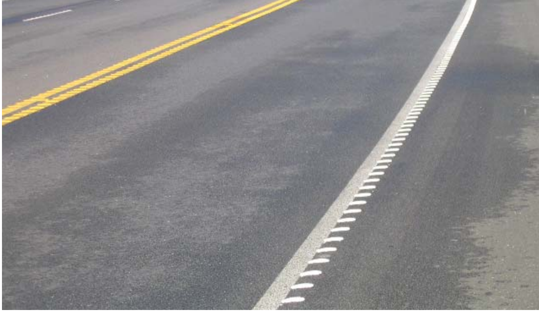
Figure 3.1 CAP ATP centre and edgeline treatment near Bombay; 100 mm wide line with 100mm ribs spaced at 250 mm
