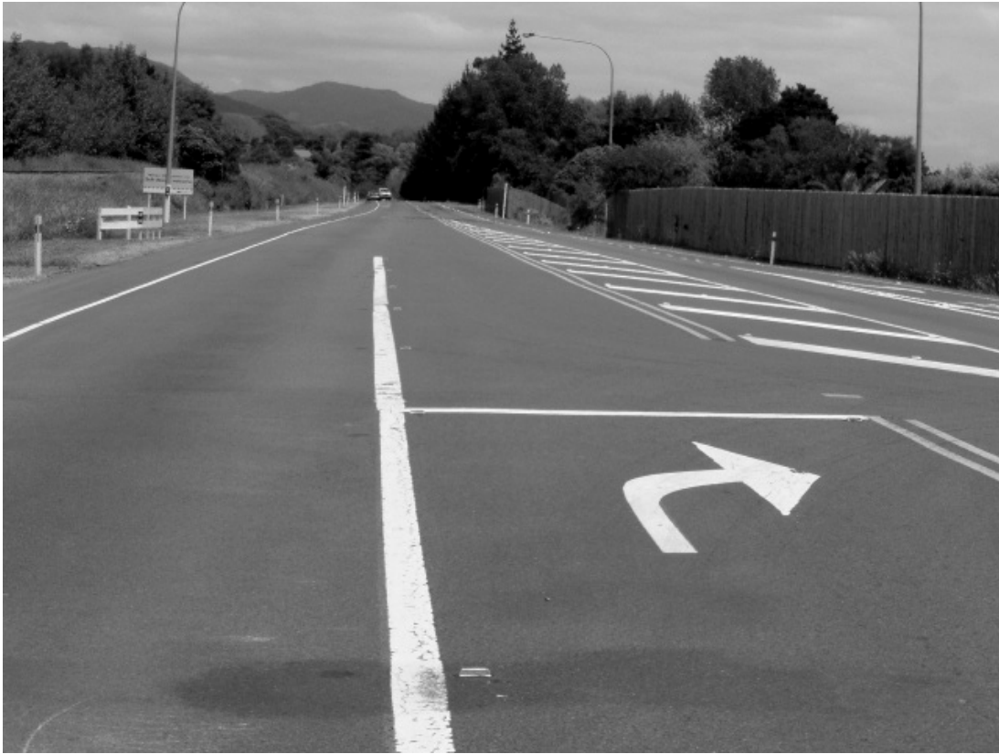
Figure 3.5 Example of right turn lanes with ATP solid lane line on the departure
