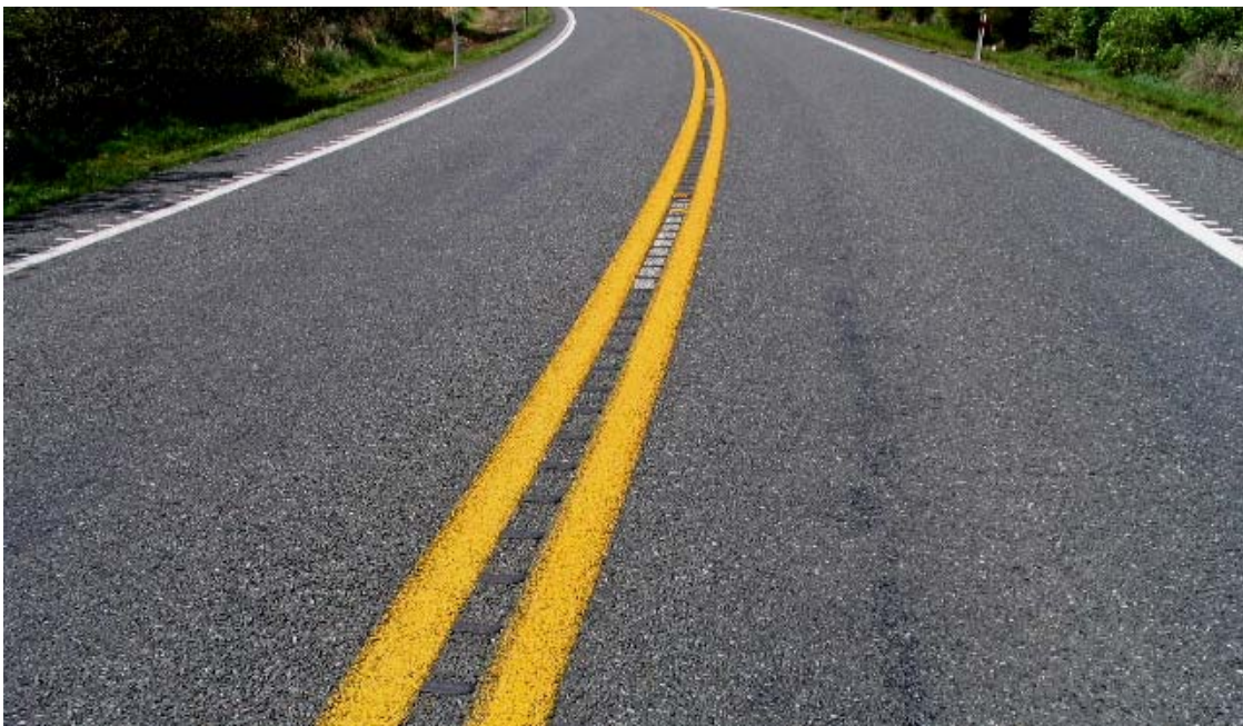
Figure 3.3 ATP double yellow centreline with black ribs and ATP edgelines, together with CAP composite edgeline and narrow shoulders
