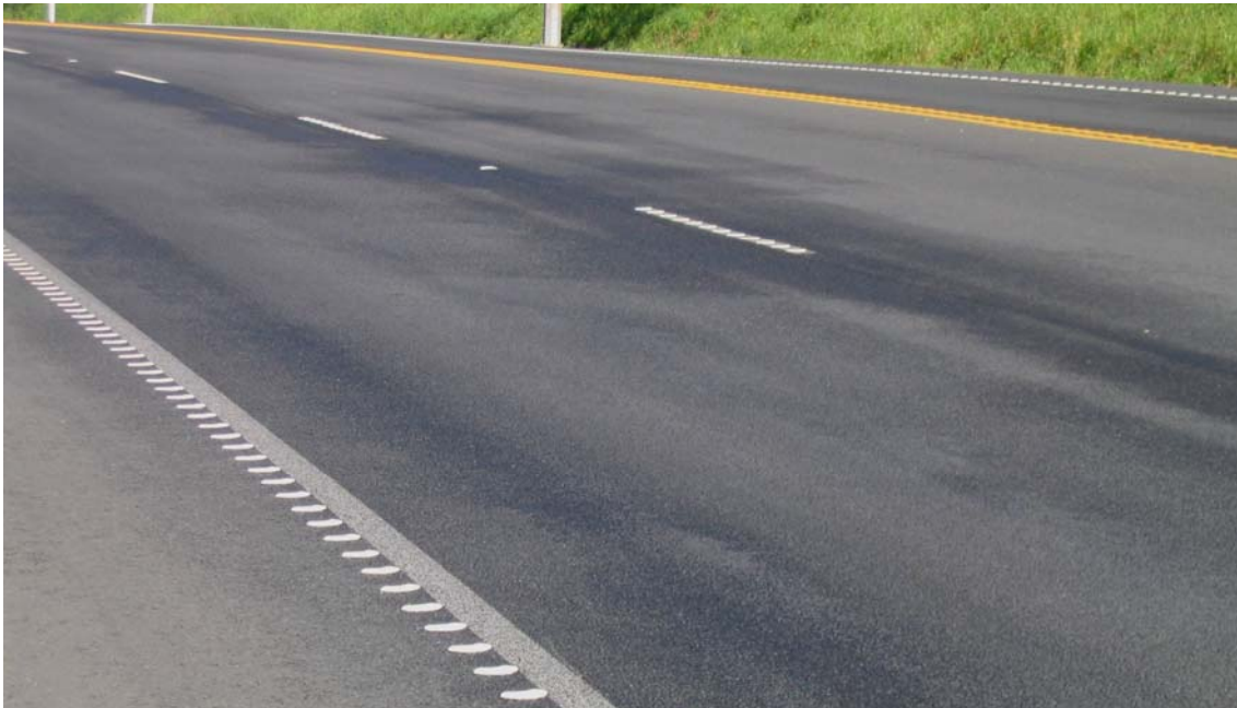
Figure 3.4 ATP edgelines placed adjacent to a painted continuous edgeline, ATP lane lines and ATP double yellow lines on SH 2 near Bombay
