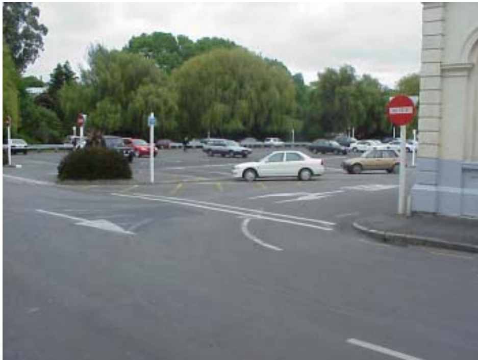
Confusing 'blacked out' right turn arrow.
