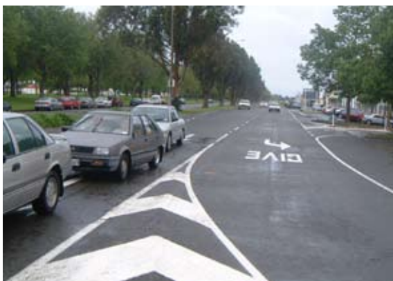
Figure 3 Captive left-turn lane with insufficient warning to motorists
