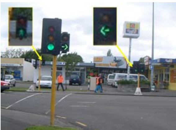
Figure 13 Walk and green left-turn arrow displayed simultaneously
