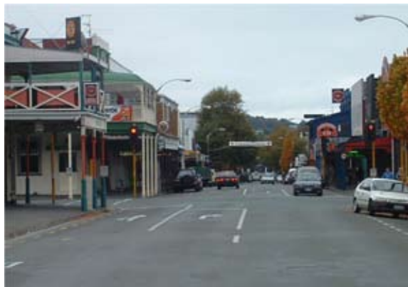
Figure 1 Offset right-turn bays (and hidden primary lantern)
