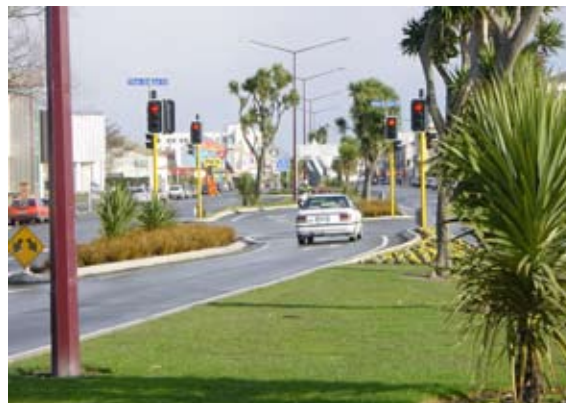
Figure 2 Right-turn bays incorporated into solid median achieving excellent forward visibility
