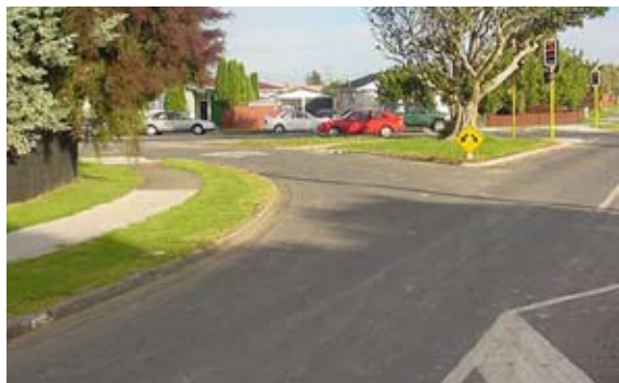
Figure 5 Pedestrian crossing around the corner – poor visibility
