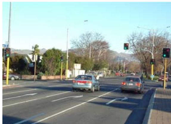
Figure 10 Fully protected right turn with the required three right-turn arrow displays
