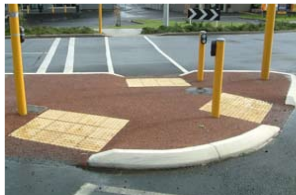
Figure 17 Use of stub post for appropriate placement of pedestrian call box adjacent to the pram crossing 1
