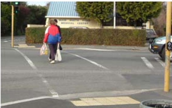
Figure 14 Bad practice of providing a crosswalk to the right of the side street at a T intersection without pedestrian protection
