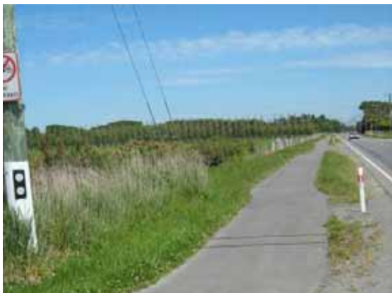
Figure A1 Typical off-road path counting installation
