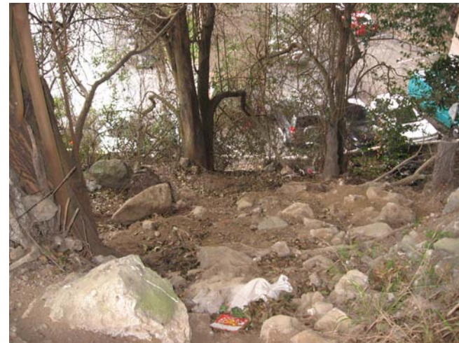
MODIFIED BASALT FLOW BENEATH NEWMARKET VIADUCT AT GILLIES AVENUE END
