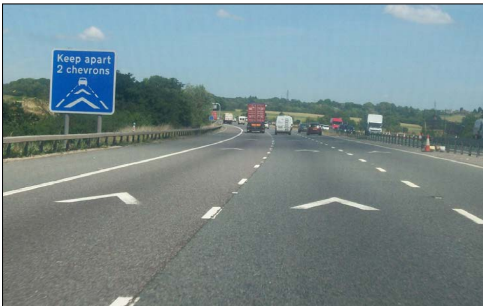
Figure 7.5 Chevron markings in the UK to encourage safer following distances (Glen Koorey)
